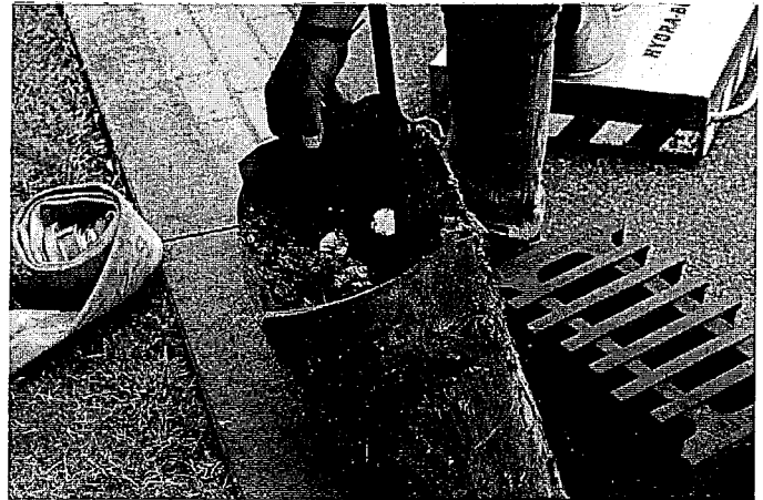
Debris from storm drains and catch basins should be collected and disposed of according to best practices and local regulations.
